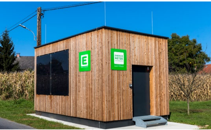
This "urban box" houses the community storage system, photo: Energie Steiermark/icon
