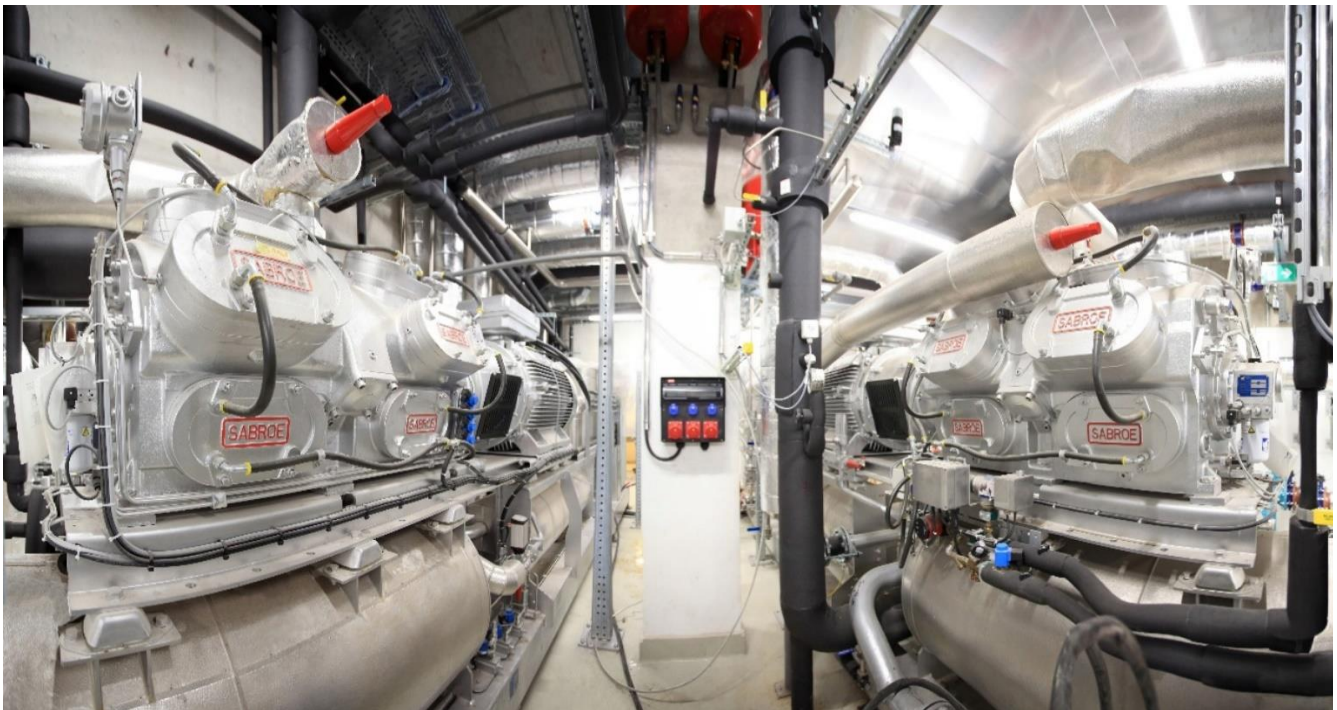
Figure 14: Heat pump system at spa Vienna (Source Klimafonds / Krobath)
