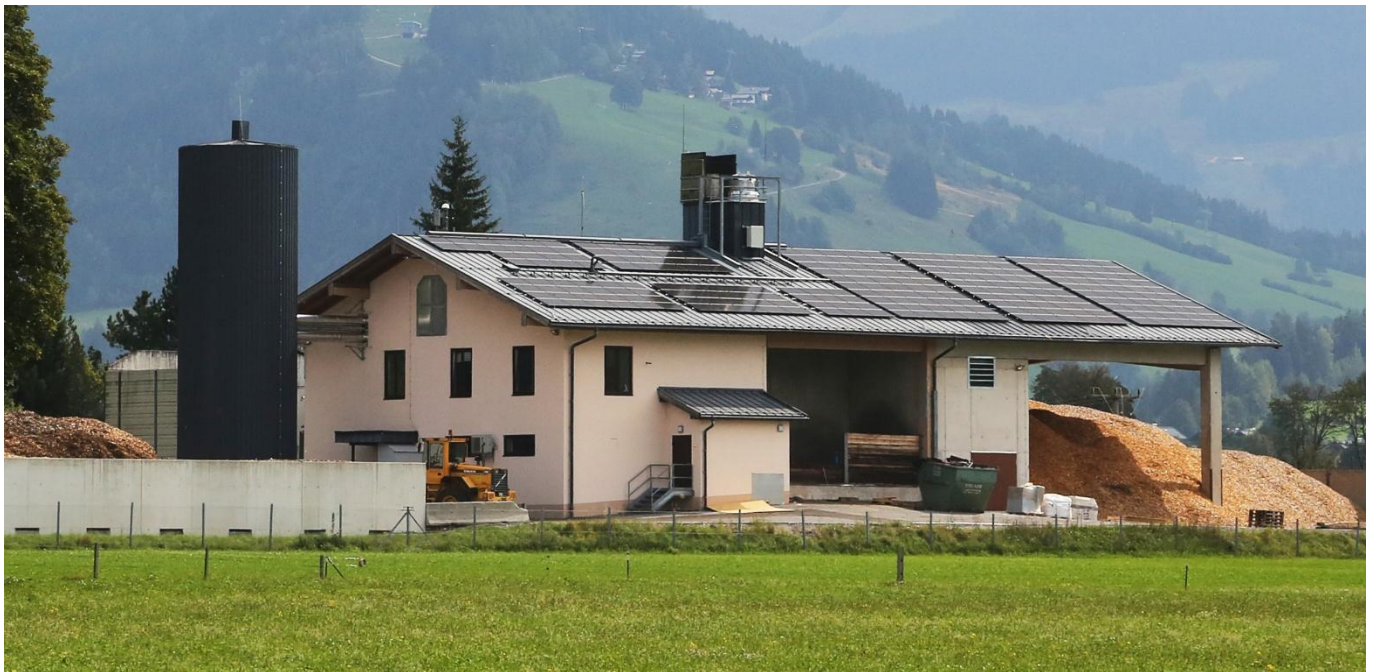
Figure 12: DH plant in Saalfelden. Source: Klimafonds / Krobath
