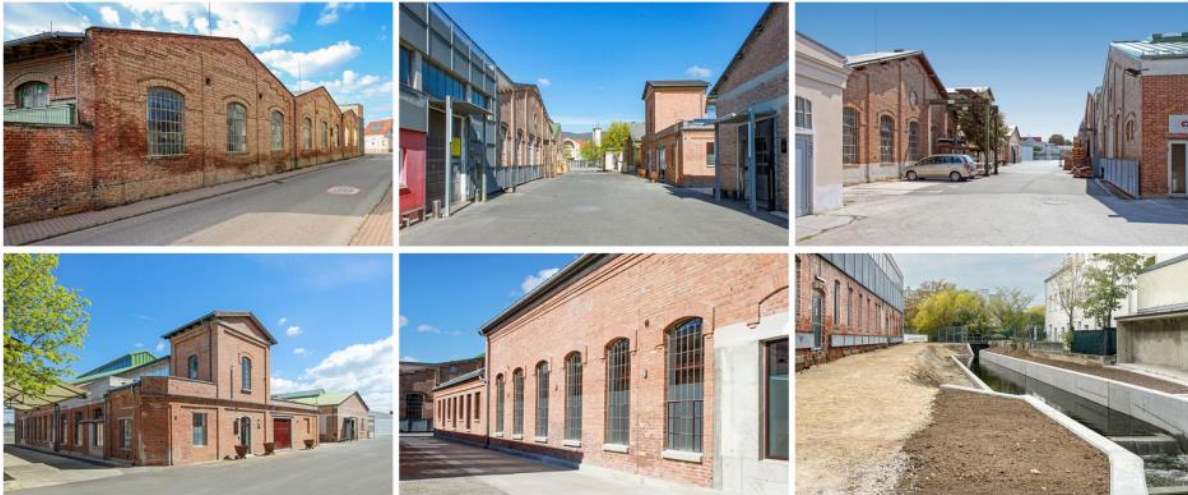
Figure 4: Existing building stock at Werk Möllersdorf. Source: Kallinger Projekte
